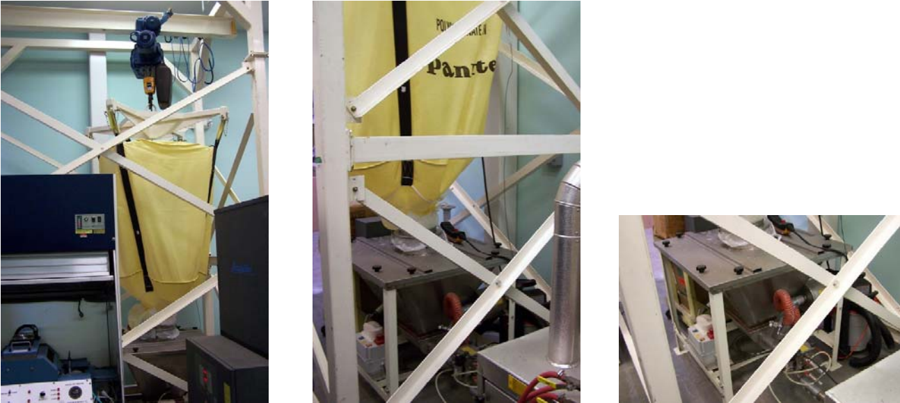
Frame not available, SS takeoff box and Piovan drying system with built in loading system all part of system.
